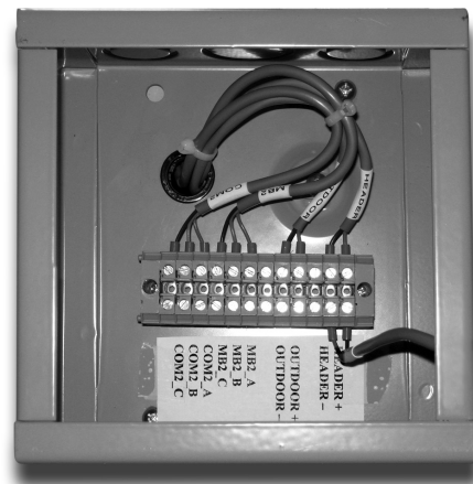
FIGURE 15. LOW VOLTAGE CONTROL WIRING
